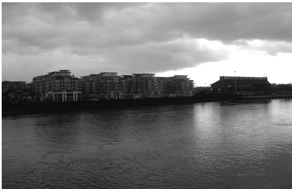
Figure 3. Wandsworth Riverside: the Riverside West development (left) and the neighbouring refuse facility (right)
